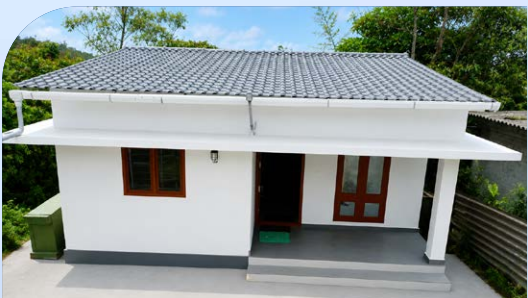
House of Vanitha, Peerumedu, Idukki
